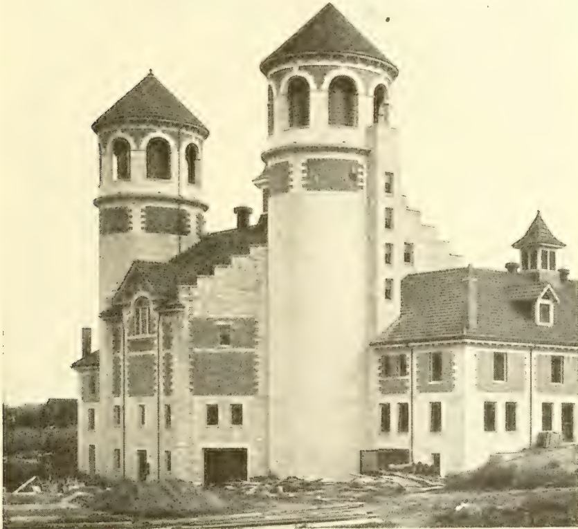
Two Decorative Silos of Ideal Blocks on the Barber Estate, Barberton, Ohio
